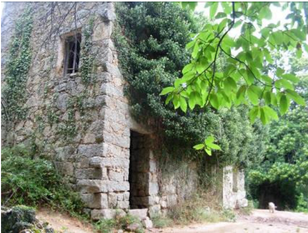
Photo 7 - YC : Abandoned Village of Tasso, municipality of Marignana
